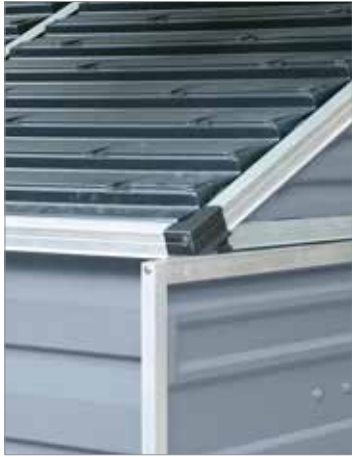
Aluminum frame and shingled roof
